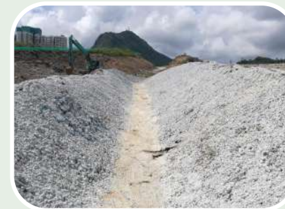
Temporary catchment channel for diversion of stormwater
