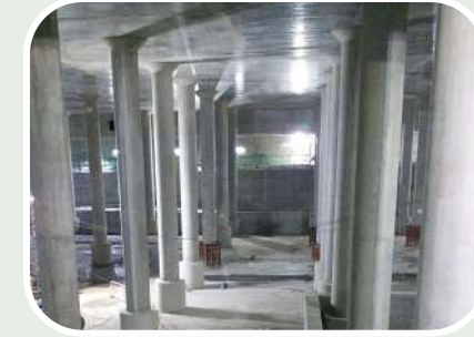
Underground Stormwater Retention Tank with 60,000m³ storage capacity
